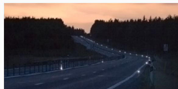
The E4 Motorway Luleå in the northern part of Sweden with LED-Mark
