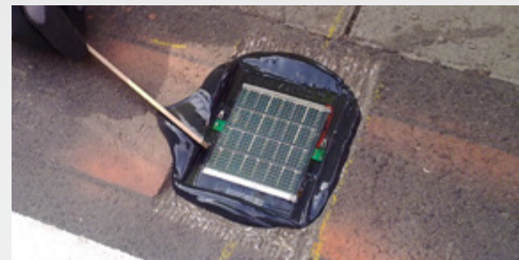
LED-Mark milled into the surface and glued on
